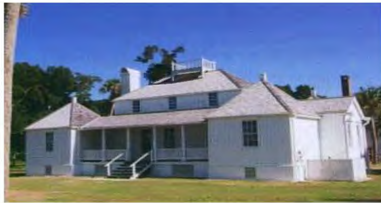
The walls of the old plantation house on Fort George Island have stood for over 200 years.
