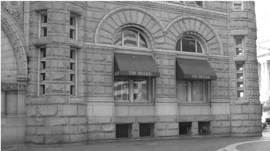
FIGURE 32: Windows North-west Pavilion, 2012. Photo Courtesy of OLBN Inc.
