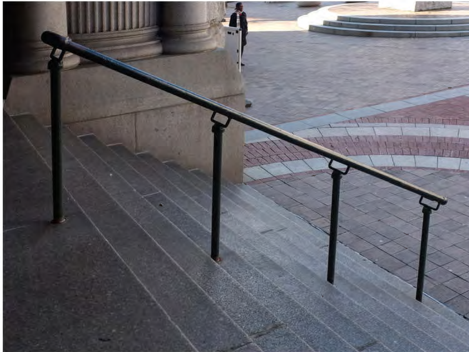
FIGURE 95: North Portico Staircase Railing, 2012. Photo Courtesy OLBN Inc.
