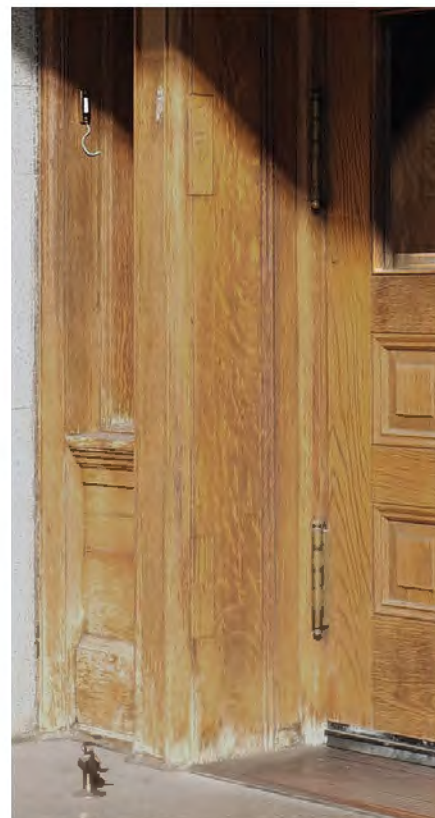
FIGURES 62 & 63: Door and Frame Condition, 2012. There are signs of weathering, particularly near the bottom the doors, where water can splash on the surfaces. . Photos Courtesy OLBN Inc..
