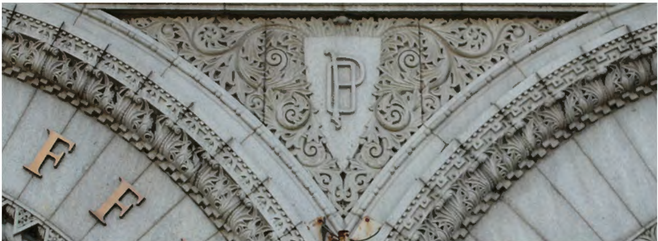
FIGURE 55: Pennsylvania Avenue Portico Spandrel, 2012. Photo Courtesy OLBN Inc.
