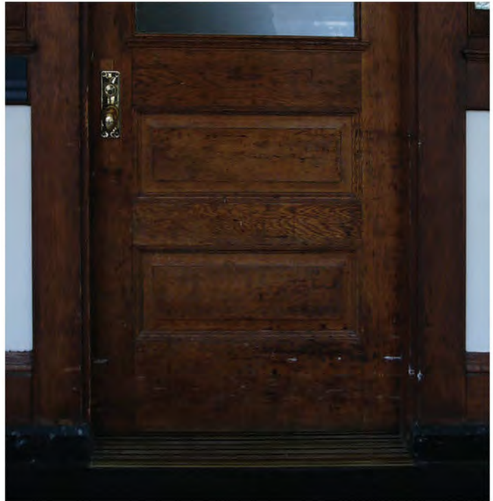
FIGURES 71 & 72: Condition of the Lower Sections of Some of the Doors' Rails and Jamb, lining the Cortile Corridor, 2012. Photos Courtesy OLBN Inc.
