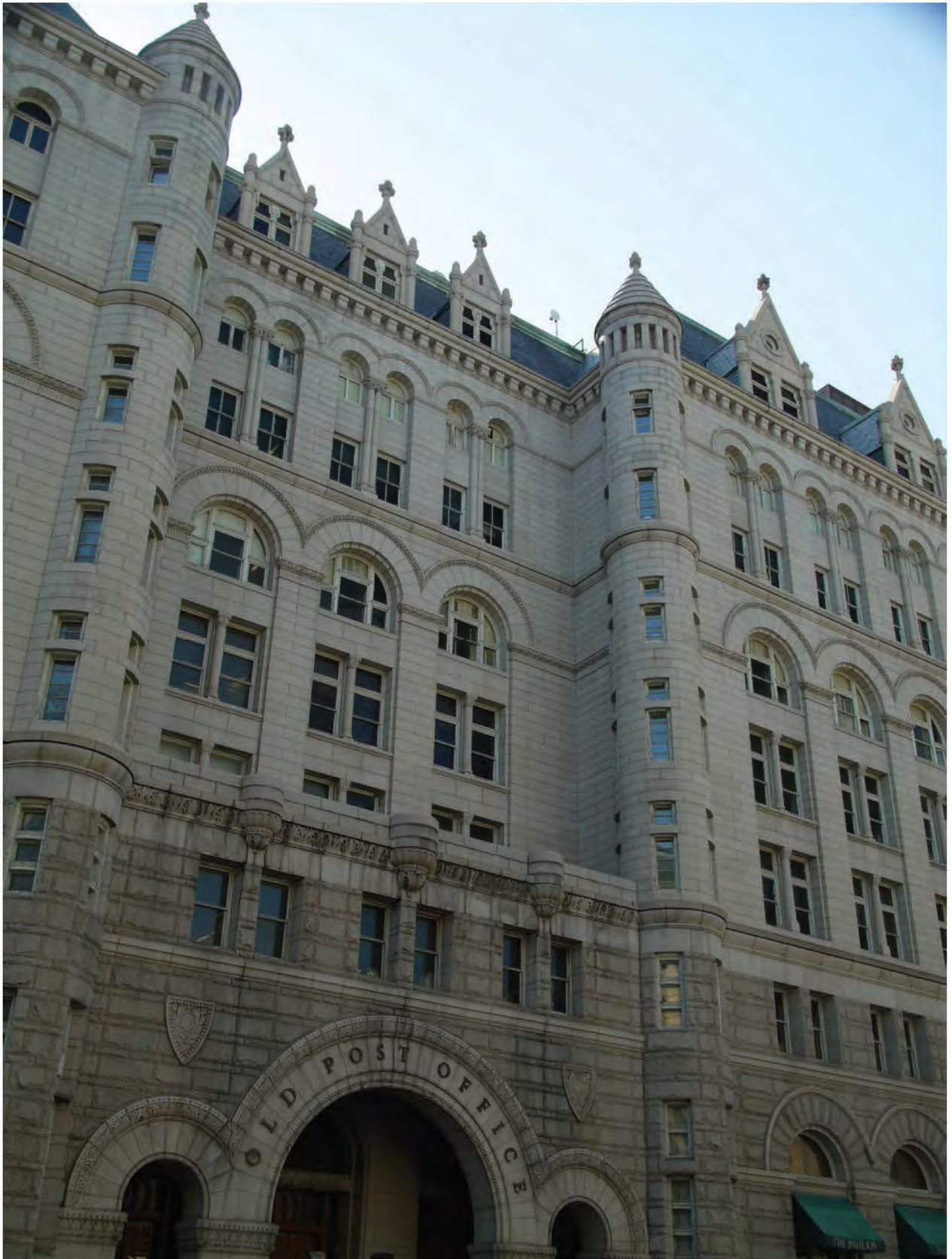
FIGURE 17: Partial View of the 12th Street Elevation of the Old Post Office Looking South, 2012. Photos Courtesy OLBN Inc.
