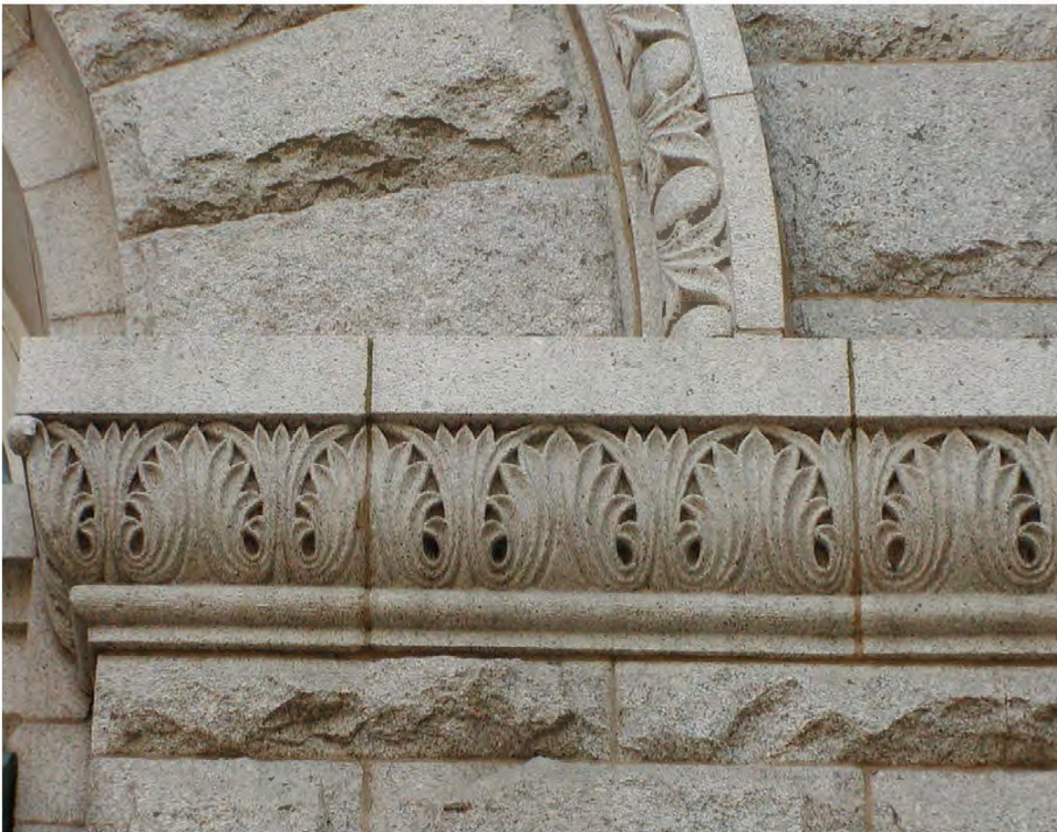
FIGURE 13: Detail of Vinalhaven Granite From the NE Turret Base, 2006. Photo Courtesy of T. McDowell.
