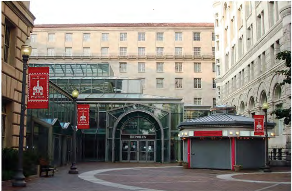
FIGURE 103: Atrium Annex, 2012. Photo Courtesy OLBN, Inc.
