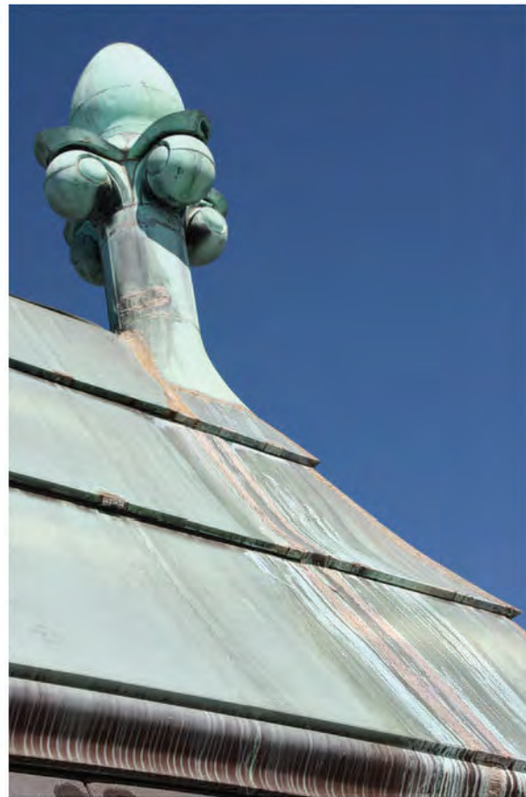
FIGURE 41: Copper Roof Finial on the Main Roof Ridge, 2012. Photo Courtesy OLBN Inc.
