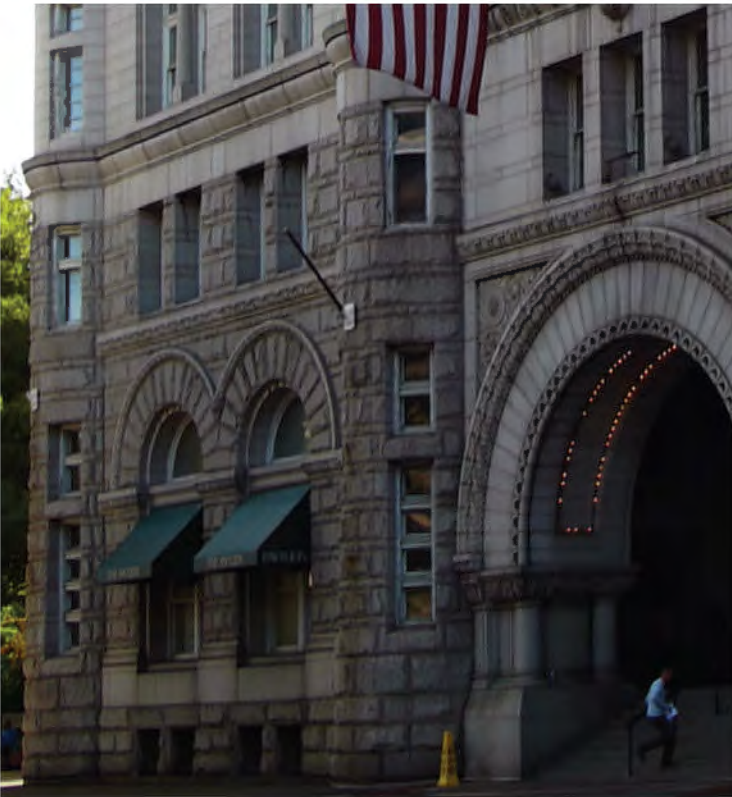
FIGURE 15: Detail of NE Building Base Openings, 2012. Photo Courtesy OLBN Inc.
