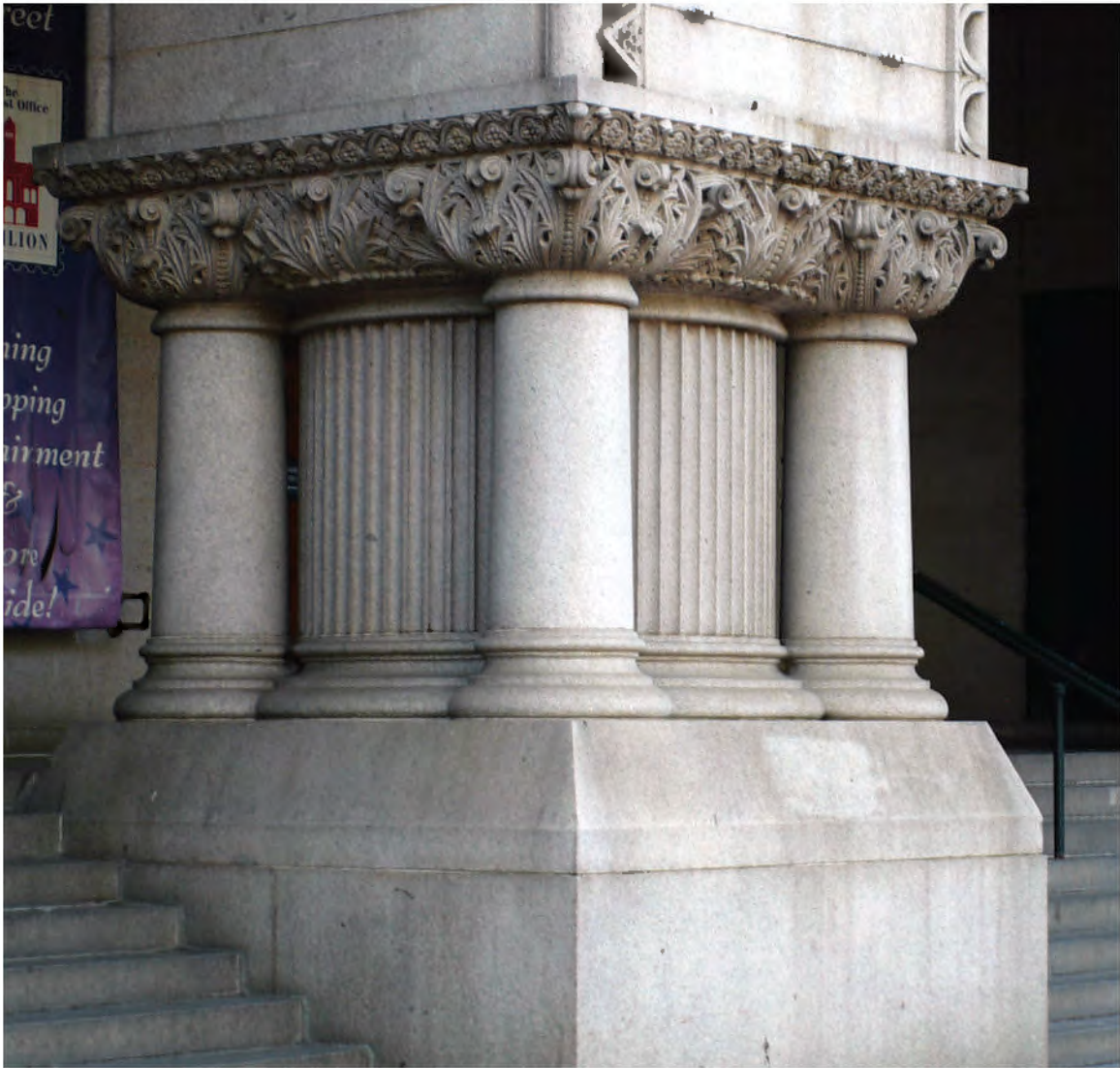
FIGURE 52: Pennsylvania Avenue Portico Pier, 2012. Photo Courtesy OLBN Inc.
