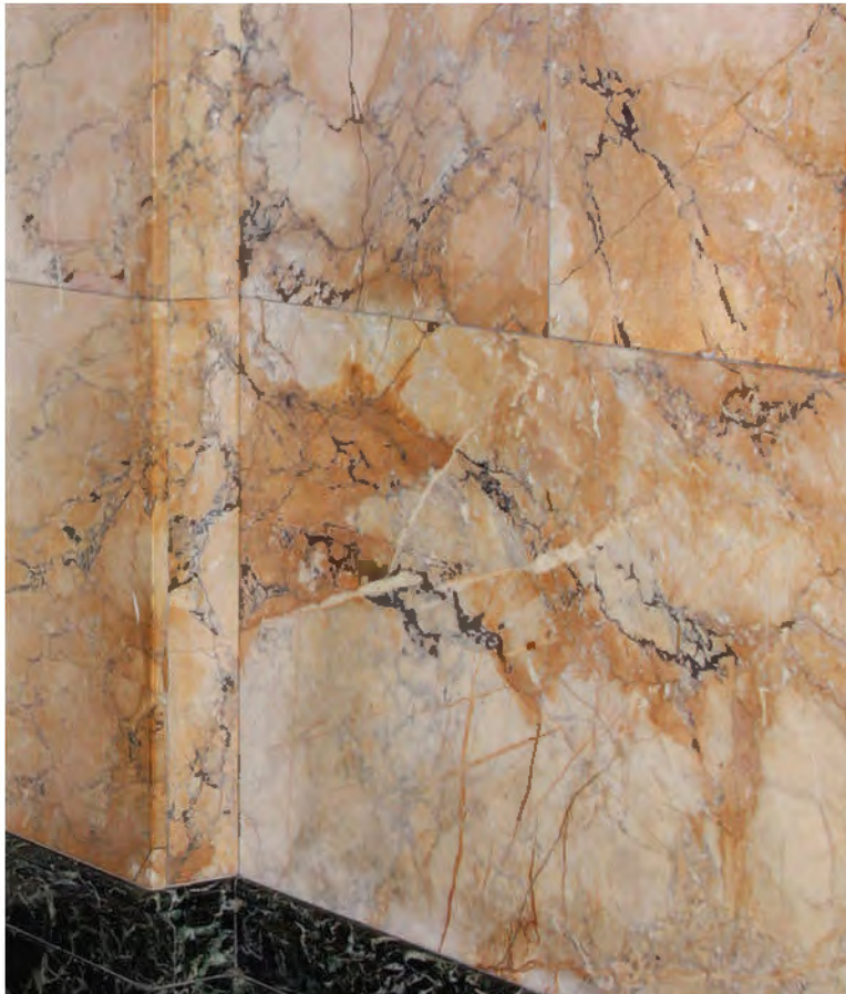
FIGURE 58: Detail of North Wall Wainscot , 2012. Image Courtesy of OLBN Inc.
