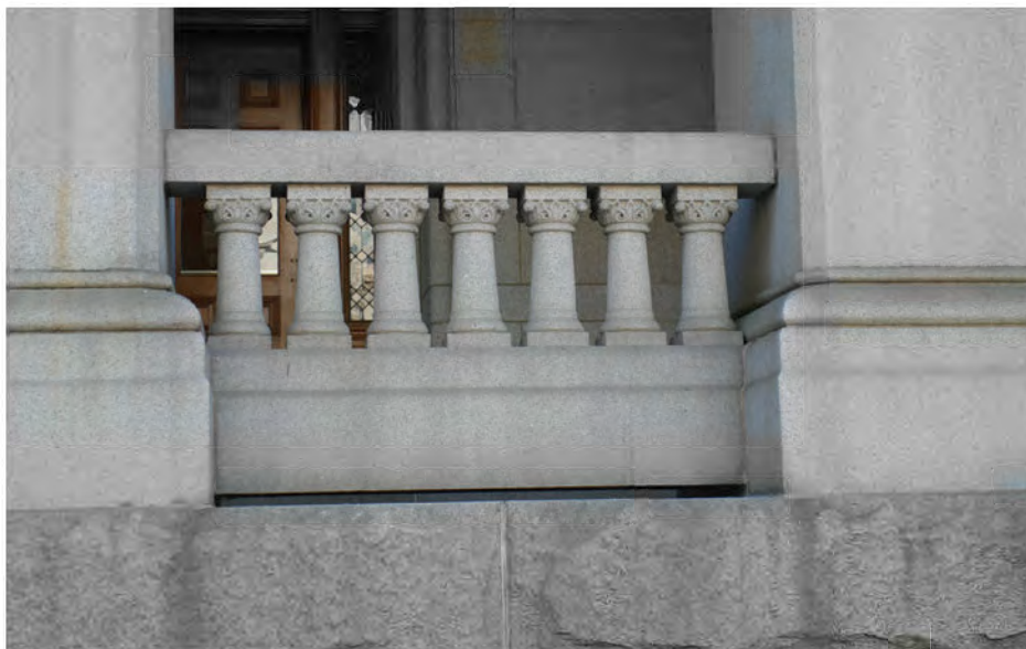
FIGURE 68: 11th Street Portico Balustrade, 2012. Photo Courtesy OLBN Inc.
