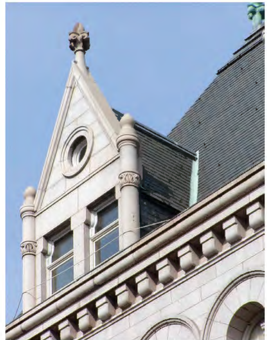
FIGURE 27: Large Dormer, 2012. Photo Courtesy OLBN Inc.
