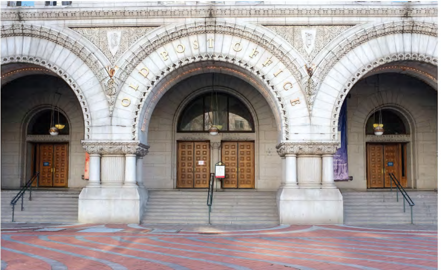
FIGURE 75: Pennsylvania Avenue Door Assemblies, 2012. Photo Courtesy OLBN Inc.
