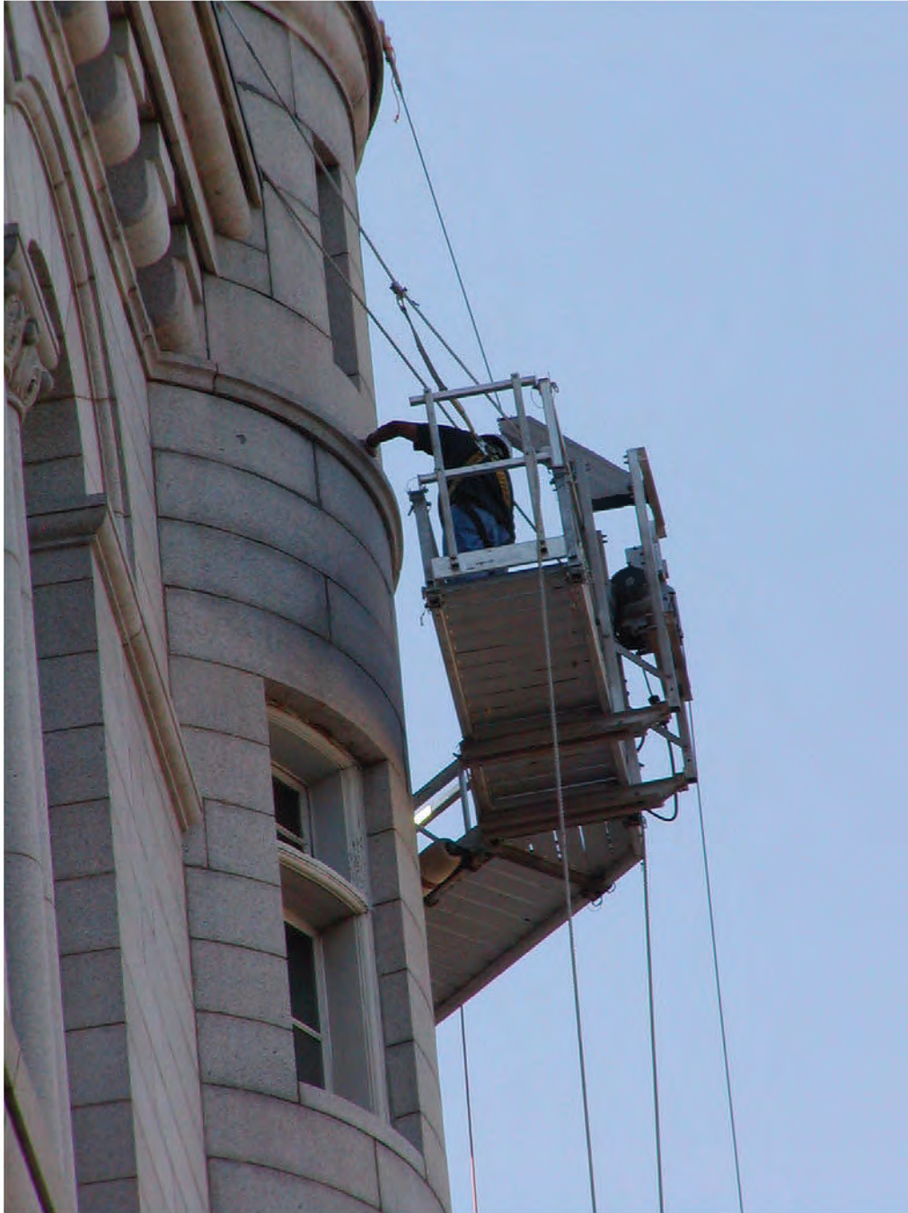
FIGURE 2: Old Post Office Repairs, 2006. Photo Courtesy of T. McDowell.
