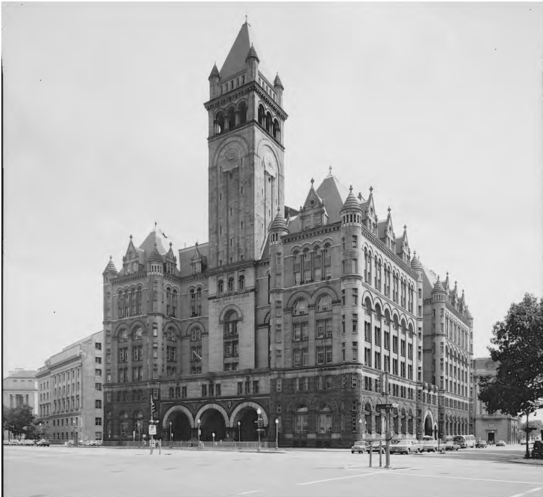
FIGURE 29: 1967 Building Exterior. Image Courtesy of the Library of Congress, Prints and Photographs Division, HABS Collection
