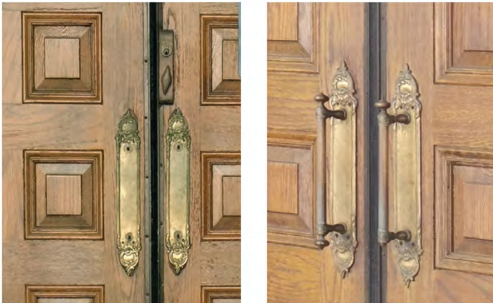
FIGURES 64 & 65: Exterior Door Hardware, Showing Different Stages Of Weathering, 2012. Photos Courtesy OLBN Inc..
