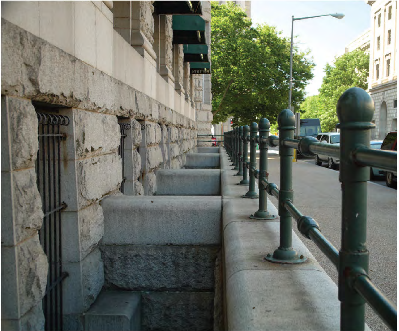
FIGURE 93: Moats and Railings 12th Street, 2012. Photo Courtesy OLBN Inc.
