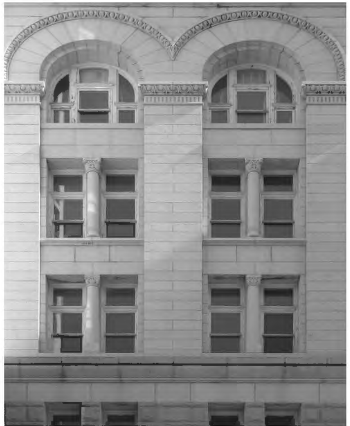
FIGURE 36: 3rd, 4th & 5th Floor Windows, 2012. Photo Courtesy of OLBN Inc.
