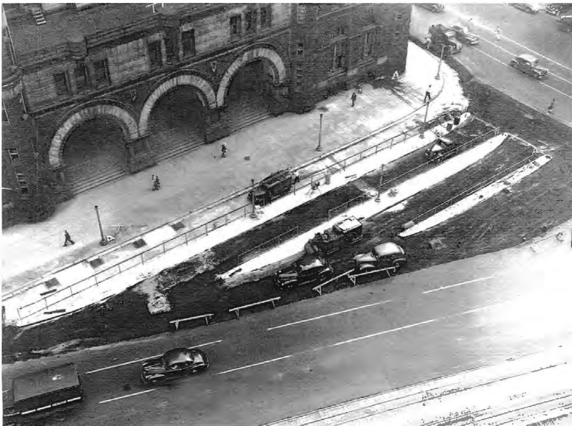
FIGURE 4: Exterior Aerial View of the Old Post Office with Bus, 1940s. Image Courtesy of the Martin Luther King, Jr. Memorial Library, Washingtoniana Collection
