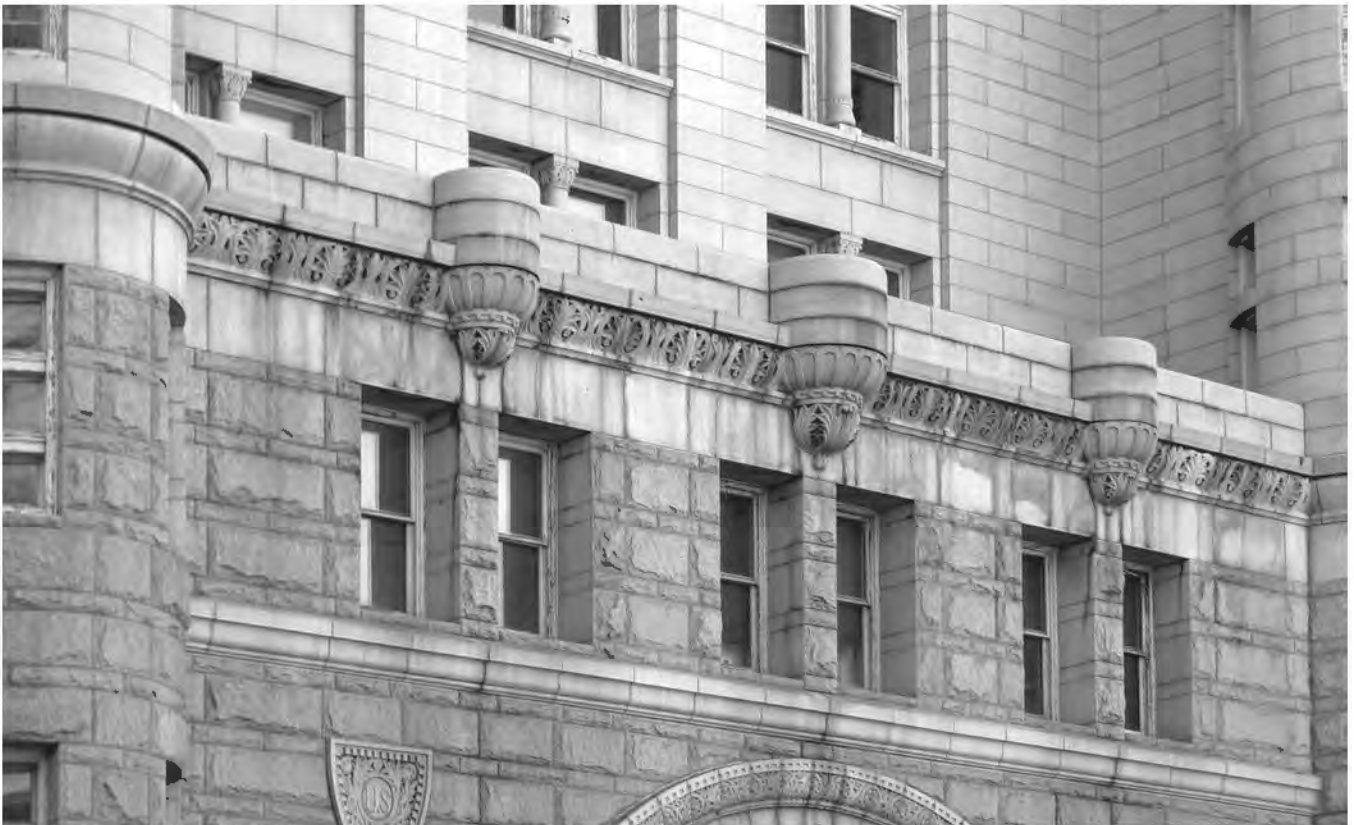
FIGURE 34: Detail 2nd Story Windows, 2012. Photo Courtesy of OLBN Inc.
