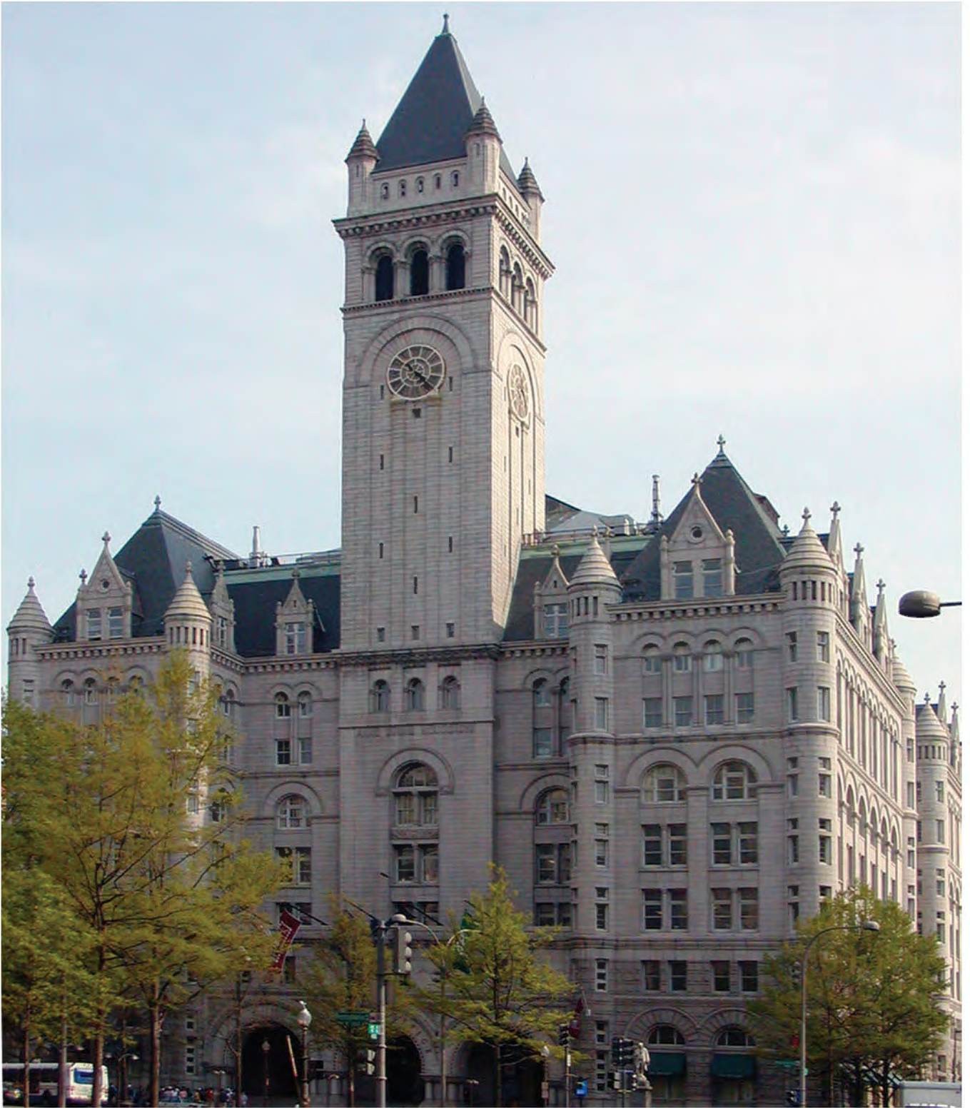
FIGURE 36: Detail of Clock Tower, 2006. Photo Courtesy T. McDowell.
