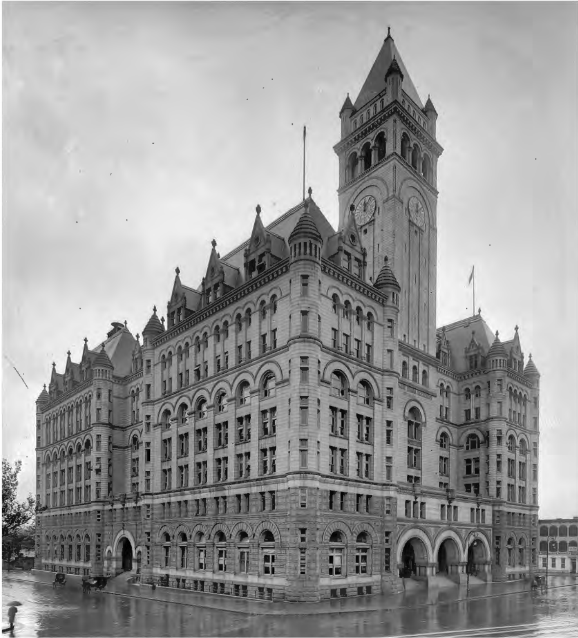
FIGURE 12: Exterior View of North-East Elevations, 1908. Image Courtesy Library of Congress, Prints and Photographs Division, Washingtoniana Collection
