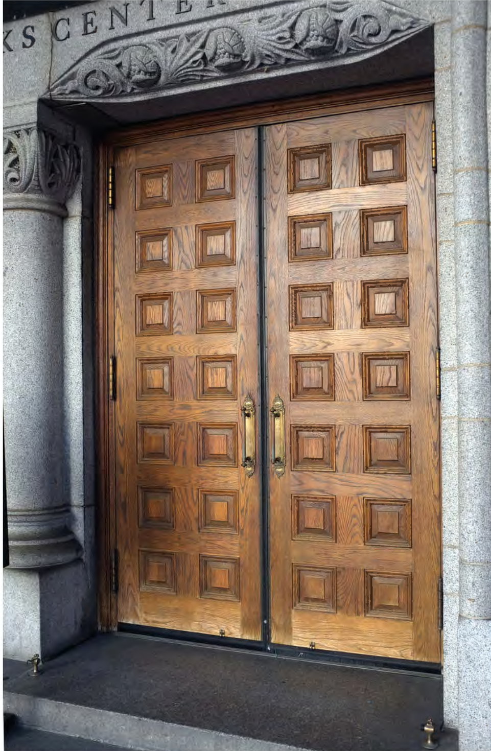
FIGURE 76: Pennsylvania Avenue Central Door Assemblies, 2012. Photo Courtesy OLBN Inc.
