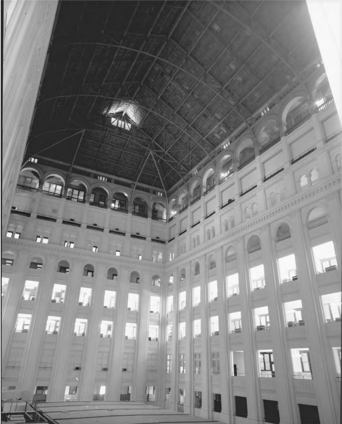
FIGURE 31: 1967 Building Interior. Image Courtesy of the Library of Congress, Prints and Photographs Division, HABS Collection
