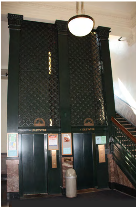
FIGURE 12: NW Elevator Cages, 2012. Photo Courtesy OLBN Inc.
