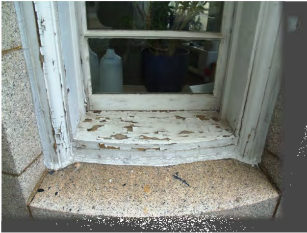
FIGURES 57 & 58: Windows Failing Paint, 2012. Photos Courtesy OLBN Inc..
