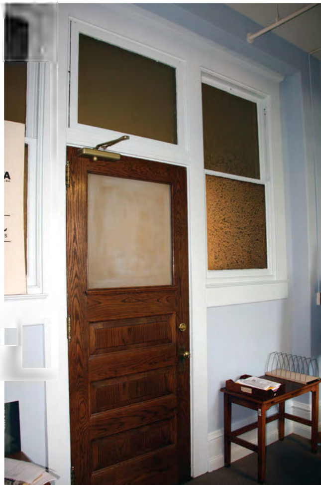
FIGURE 8: 7th Floor Typical Office. Detail. Image OLBN Inc, 2012
