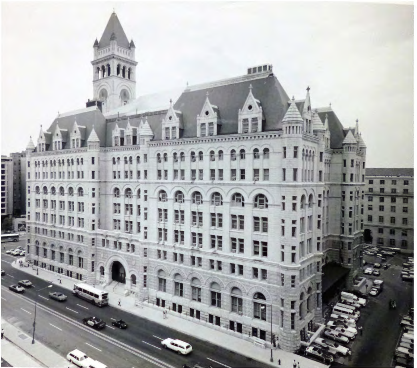
FIGURE 43: August 10, 1977 Photograph of the Washington D.C. Post Office. Image Courtesy of GSA-NCR Technical Resource Center.
