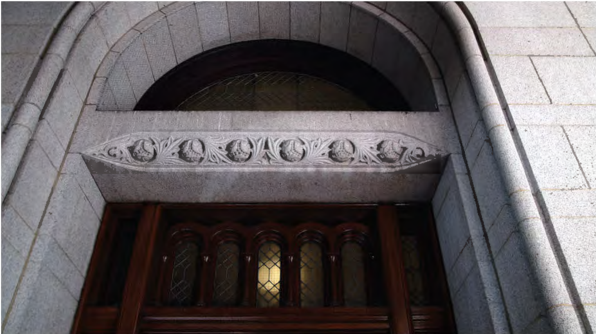
FIGURE 72: 12th Street Archway Lintel. Photo Courtesy OLBN Inc.
