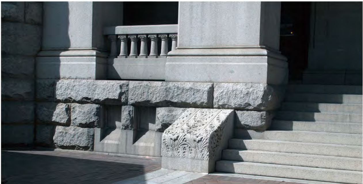
FIGURE 21: East Entrance Detail, 2012. Photo Courtesy of OLBN Inc.
