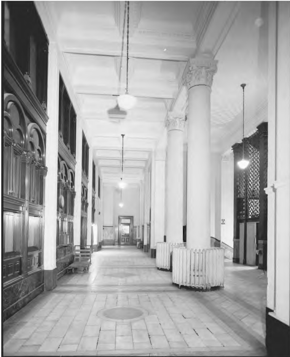
FIGURE 64: HABS photograph of the Eleventh Street corridor and stair hall, 1967. Image Courtesy of the Library of Congress, Prints and Photographs Division, HABS Collection
