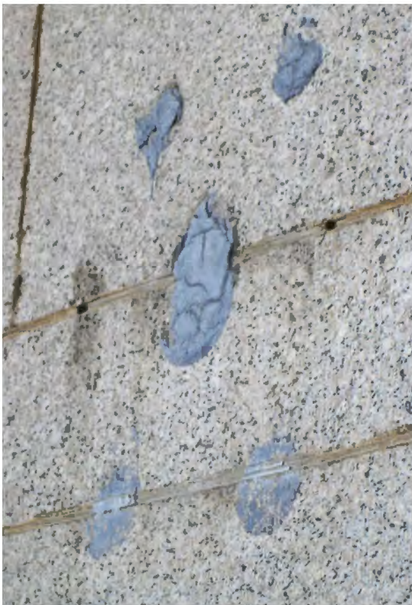
FIGURES 27, 28 & 29: Ferrous Anchors That Have Not Been Removed From The Masonry Wall Can Deteriorate The Granite, 2012. Photos Courtesy OLBN Inc.
