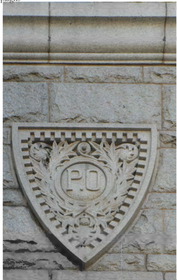
FIGURE 64: 11th Street Portico Crest, 2012. Photo Courtesy OLBN Inc.
