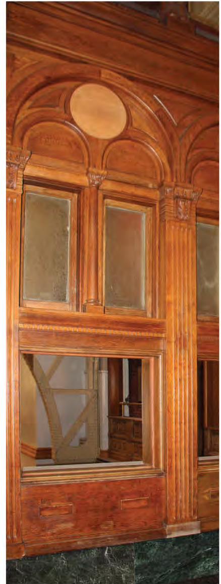
FIGURE 67: Original Oak Screen Wall from the 12th Street Corridor, 2012. Photos Courtesy OLBN Inc..
