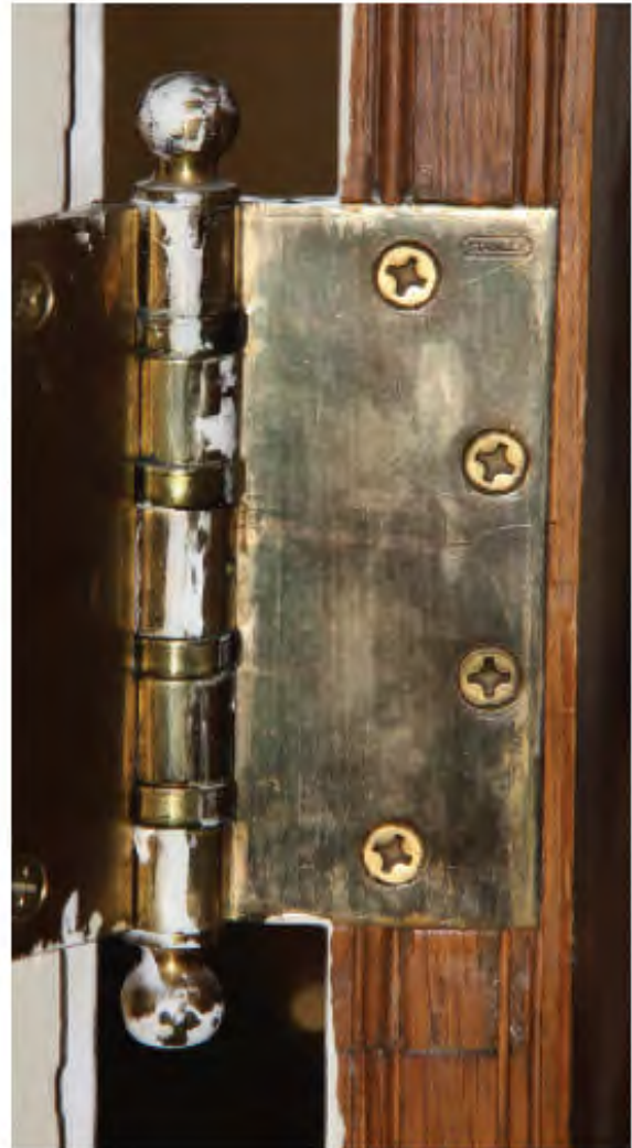
FIGURES 35, 36 & 37: Interior Features Showing Over Paint, 2012. Photos Courtesy OLBN Inc.
