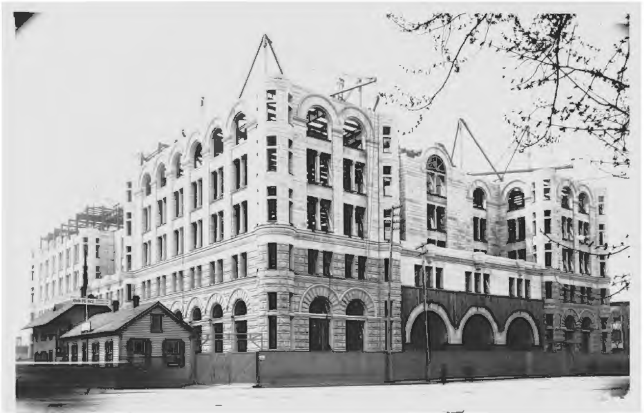
FIGURE 51: Post Office under construction; structural skeleton can be seen behind stone façade. Image Courtesy of the Library of Congress, Prints and Photographs Division, HABS Collection
