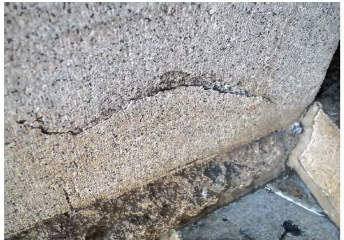
FIGURES 16, 17, 18 & 19: 11th Street Portico Cracks, Breaks & Spalling, September 2012. Photo Courtesy OLBN Inc.
