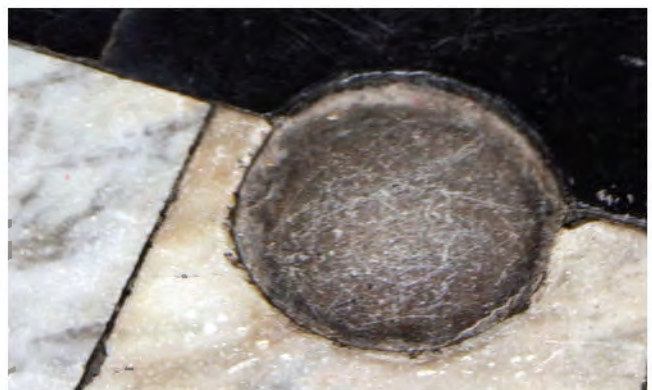
FIGURES 76, 77, 78 & 79: Different Types of Mechanical Damage Inflicted on the Marble Floor, 2012. Photos Courtesy OLBN Inc..
