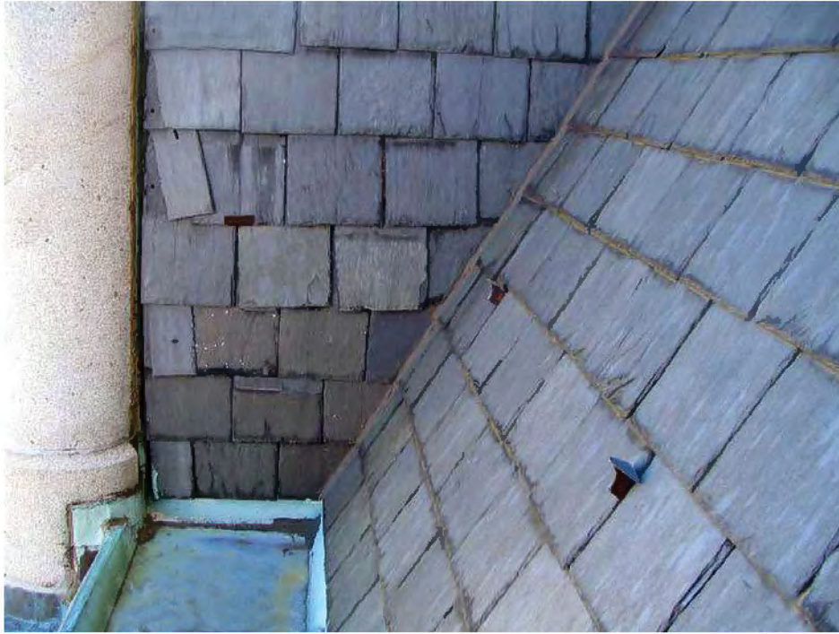
FIGURE 104: Roof, 2006. Photo Courtesy T. McDowell
