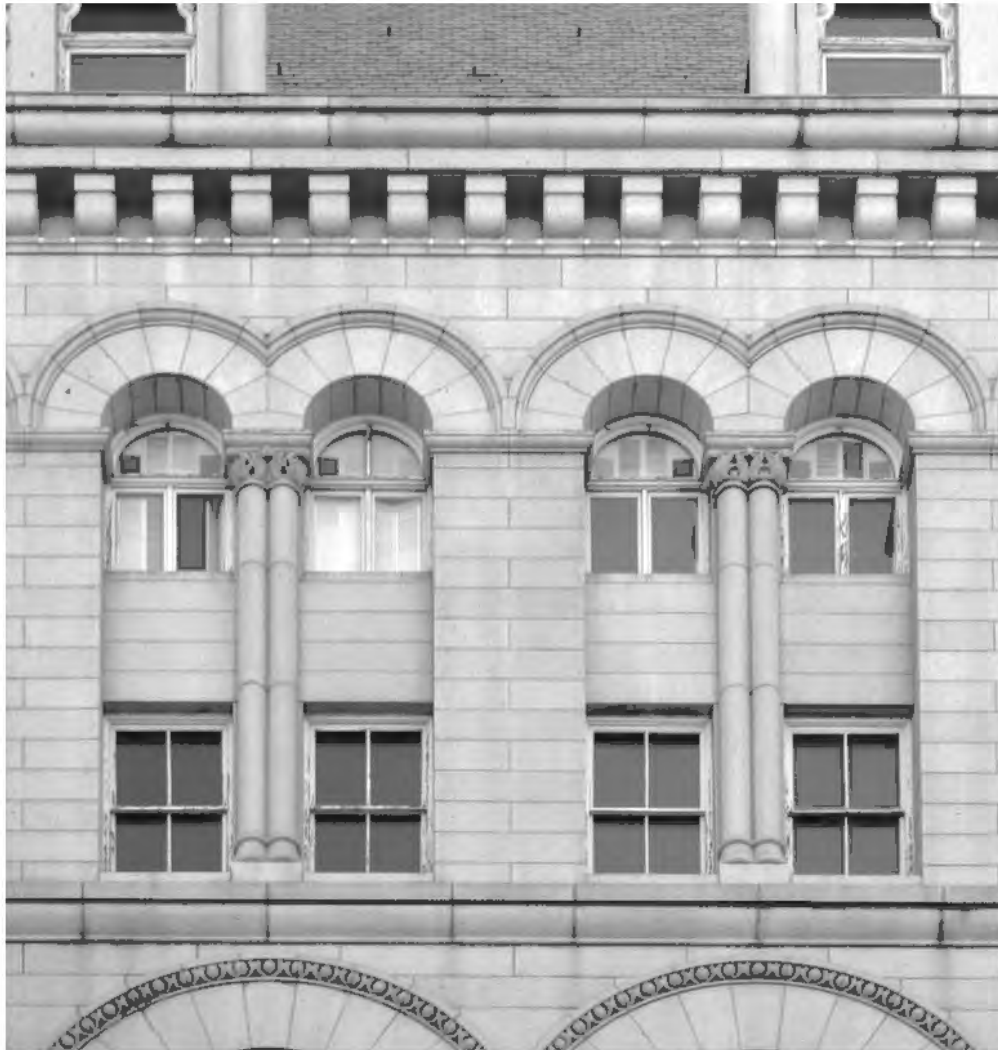
FIGURE 43: 6th & 7th Floor Windows, 2012. Photo Courtesy of OLBN Inc.
