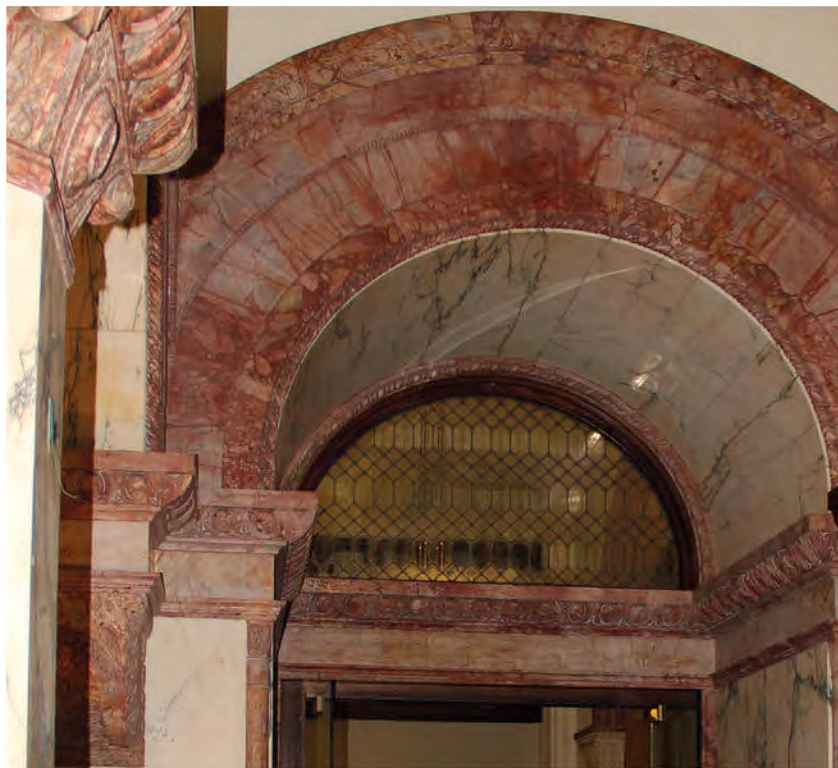
FIGURE 21: Detail of Tower Lobby Cornice/ Impost Course, 2012. Image Courtesy of OLBN Inc.
