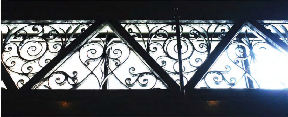
FIGURE 96: South Elevation Truss, 2012. Photo Courtesy OLBN Inc.
