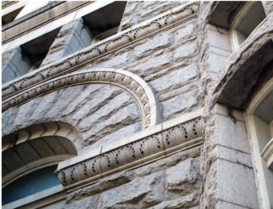
FIGURE 17: Detail of NW Pavilion 1st Floor Impost Course and Windows Label Course, 2012. Photo Courtesy OLBN Inc.
