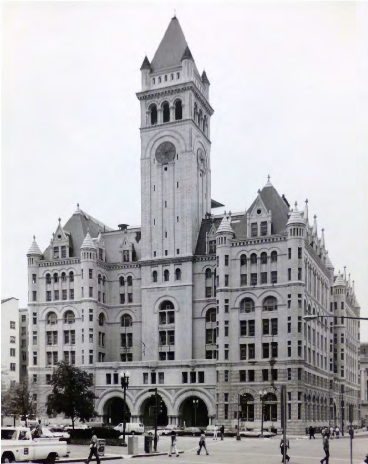
FIGURE 94: August 10, 1977 Photograph of the Washington D.C. Post Office. Image Courtesy of GSA-NCR Technical Resource Center.
