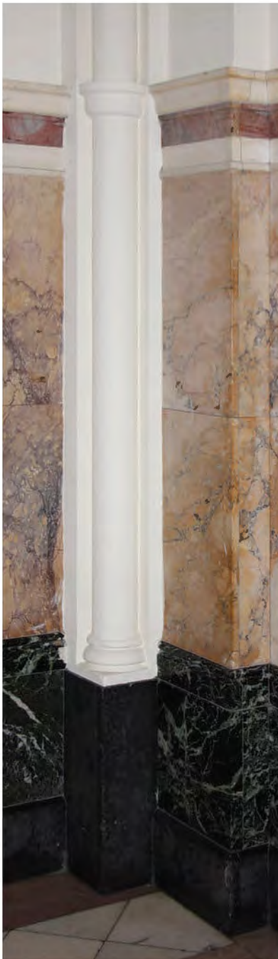
FIGURE 56 : Detail of North Wall Pilaster, 2012. Image Courtesy of OLBN Inc.
