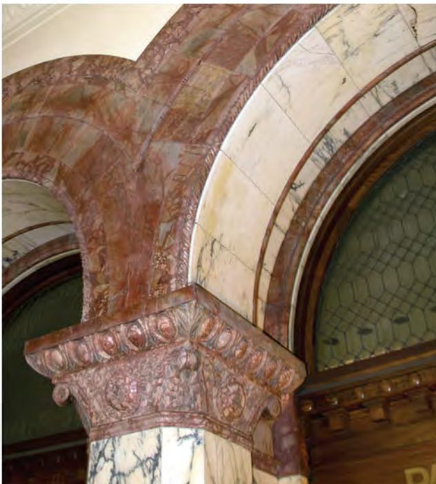
FIGURE 36: Detail of Tower Lobby South Wall, 2012. Image Courtesy of OLBN Inc.
