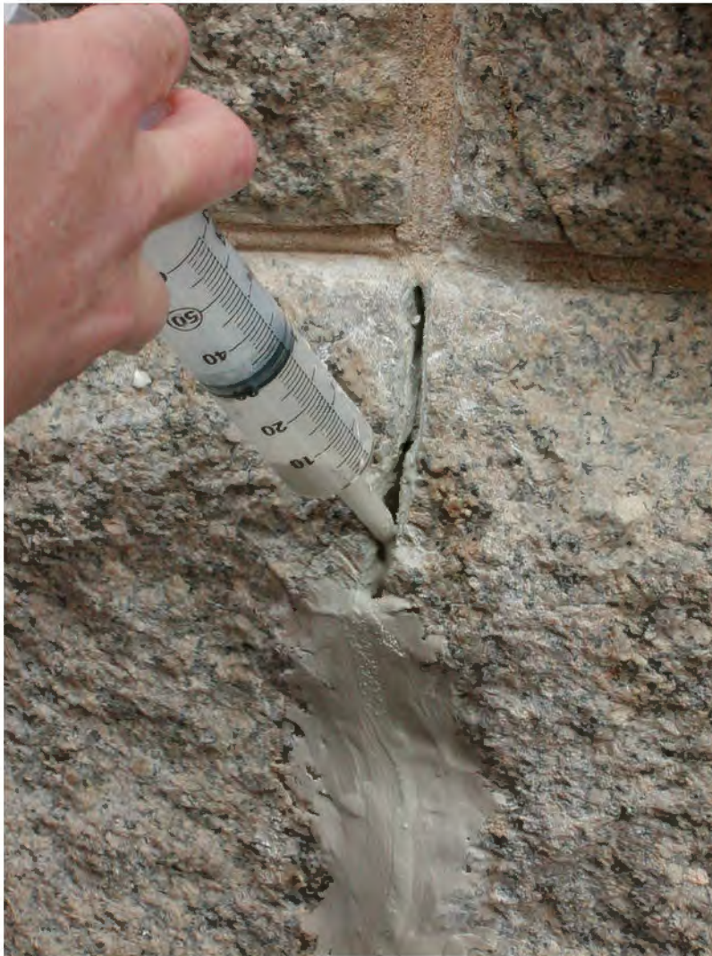
FIGURE 14: Successful Repair Campaigns, September 2006. Photo Courtesy T. McDowell
