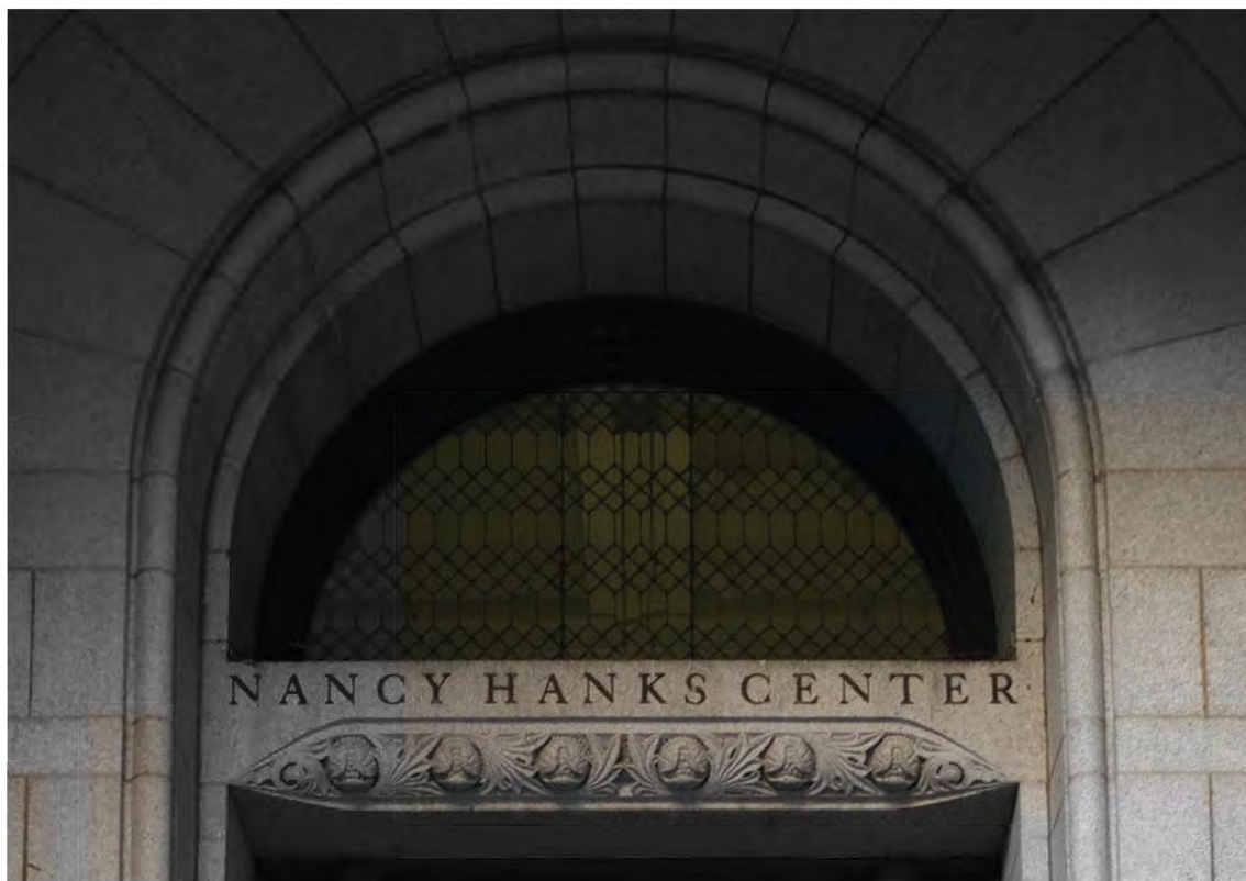
FIGURE 87: 11th Street Door Upper Transom, 2012. Photo Courtesy OLBN Inc.
