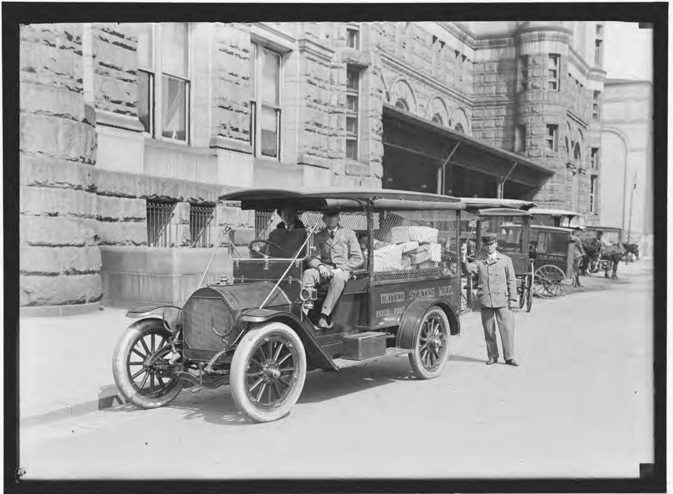
FIGURE 1: 1914 South Entrance and Postal Delivery Trucks.. Image Courtesy of the Library of Congress, Prints and Photographs Division.
