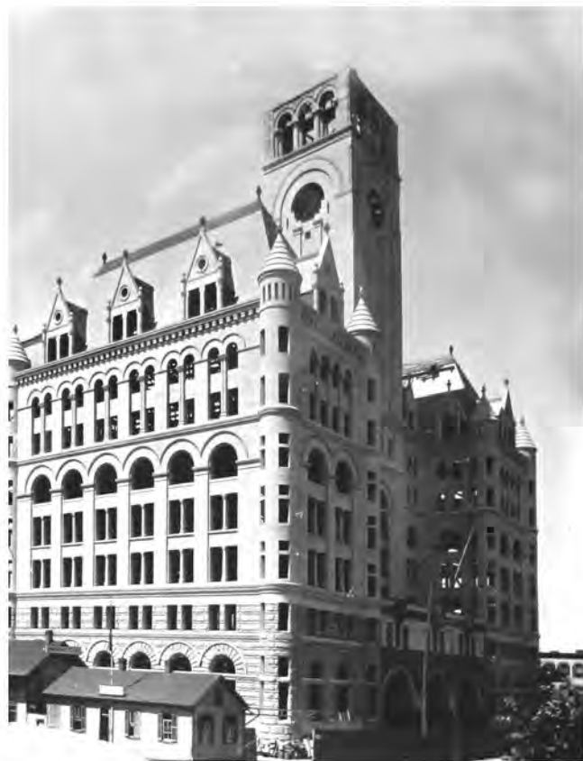
FIGURE 53: Post Office under construction; structural skeleton can be seen behind stone façade. Image Courtesy of the Library of Congress, Prints and Photographs Division, HABS Collection
