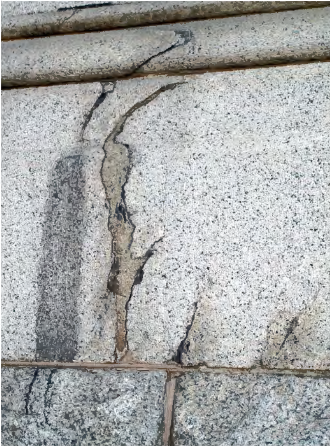
FIGURES 12 & 13: 11th Street Portico Failed Repair Campaigns, September 2012. Photo Courtesy OLBN Inc.
