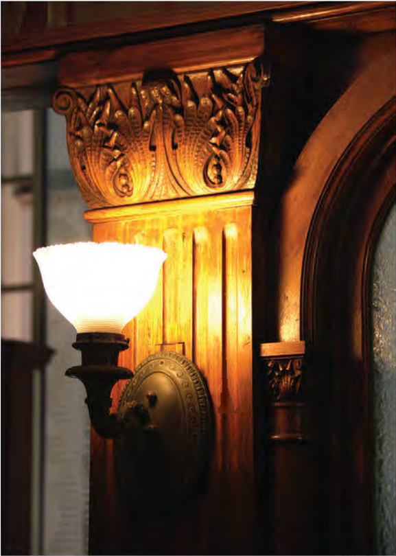
FIGURE 49: Detail of Tower Lobby Feature Wall Pilaster, 2012. Image Courtesy of OLBN Inc.
