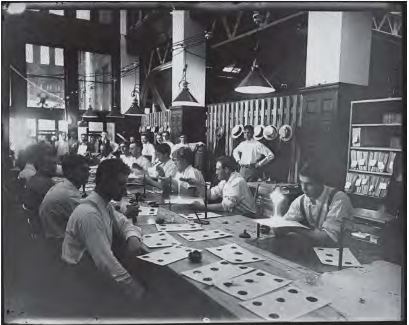
FIGURE 77: Undated Photograph of Southwest corner of Mail Workroom, Facing Northwest. Image Courtesy the Library of Congress, Prints and Photographs Division, Washingtoniana Collection. Windows at background left overlook Registry Division; trusses of workroom laylight can be seen at right.
