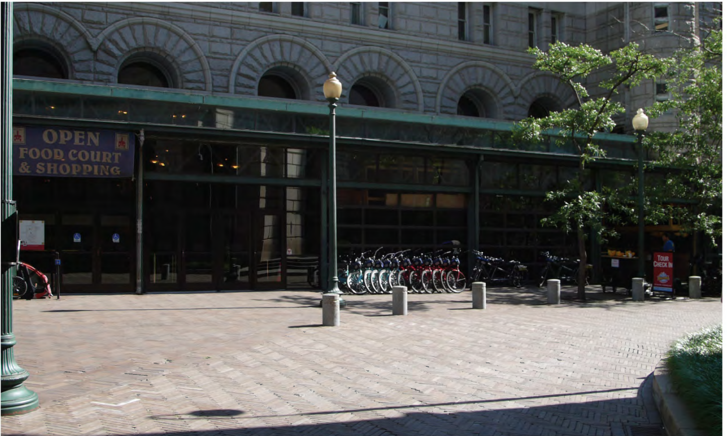
FIGURE 97: South Elevation Entrance, 2012. Photo Courtesy OLBN Inc.
