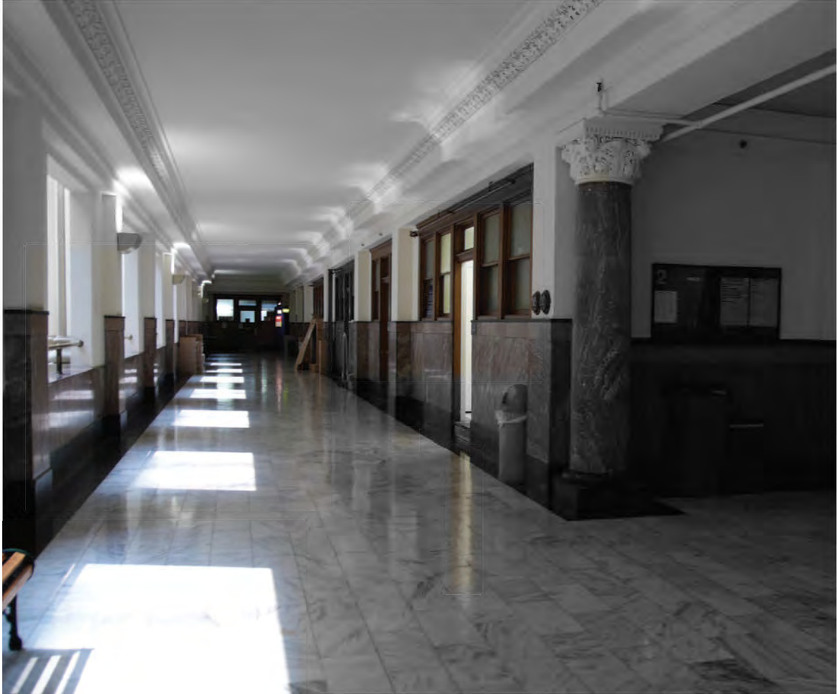
FIGURE 1: 2nd Floor West Corridor, July 2012. Photo OLBN Inc.
