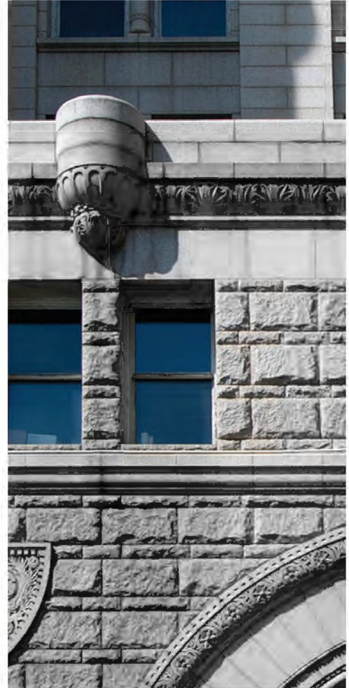
FIGURE 7: Granite Detail, 2012. Photo Courtesy of OLBN Inc.
