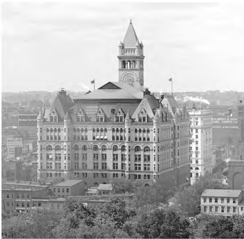
FIGURE 10: Detail of photograph showing northern façade of building, 1904 Image Courtesy of the Library of Congress, Prints and Photographs Division, Washingtoniana Collection
