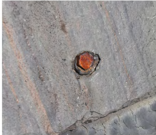
FIGURES 50 & 51: Improper Slate Repair u Face nailing the slates to the sheathing, 2012. Photos Courtesy OLBN Inc..
