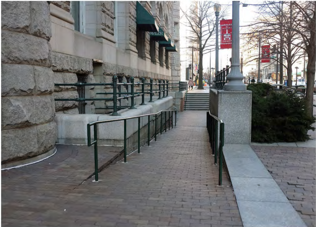
FIGURE 6: New East Entrance 11th Street, N.W., Looking North, February 2013. Photo OLBN Inc.
