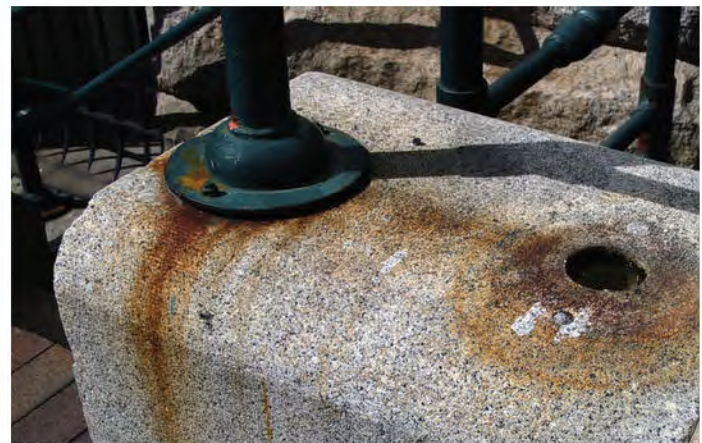
FIGURES 27, 28 & 29: Ferrous Anchors That Have Not Been Removed From The Masonry Wall Can Deteriorate The Granite, 2012. Photos Courtesy OLBN Inc.
