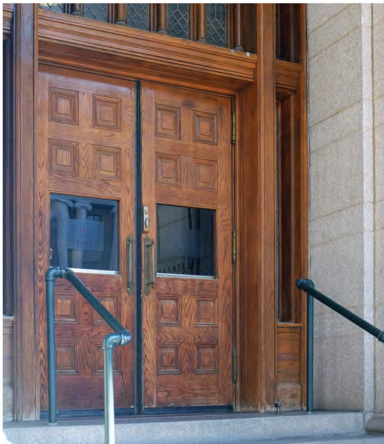
FIGURE 83: 12th Street Door Assembly, 2012. Photo Courtesy OLBN Inc.
