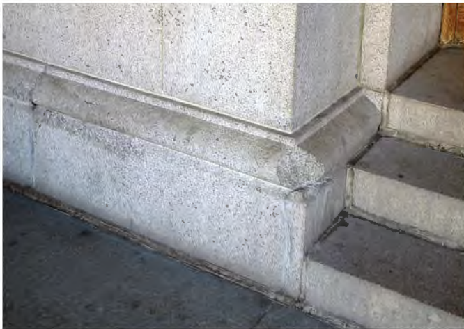
FIGURES 16, 17, 18 & 19: 11th Street Portico Cracks, Breaks & Spalling, September 2012. Photo Courtesy OLBN Inc.
