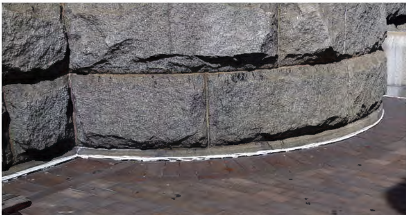
FIGURES 24, 25 & 26: Inappropriate Bituminous Joints Found Around the Perimeter of the Building, 2012. Photos Courtesy OLBN Inc.
