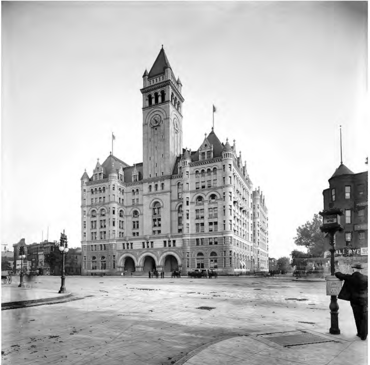
FIGURE 35: Detail of Exterior of North-East Elevations, 1905.
