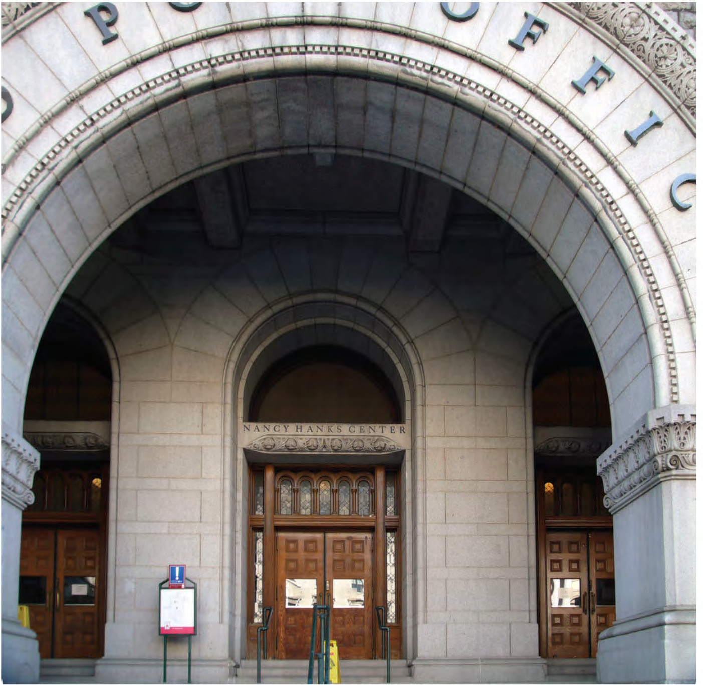
FIGURE 71: 12th Street Entrance Archways, 2012. Photo Courtesy OLBN Inc.
