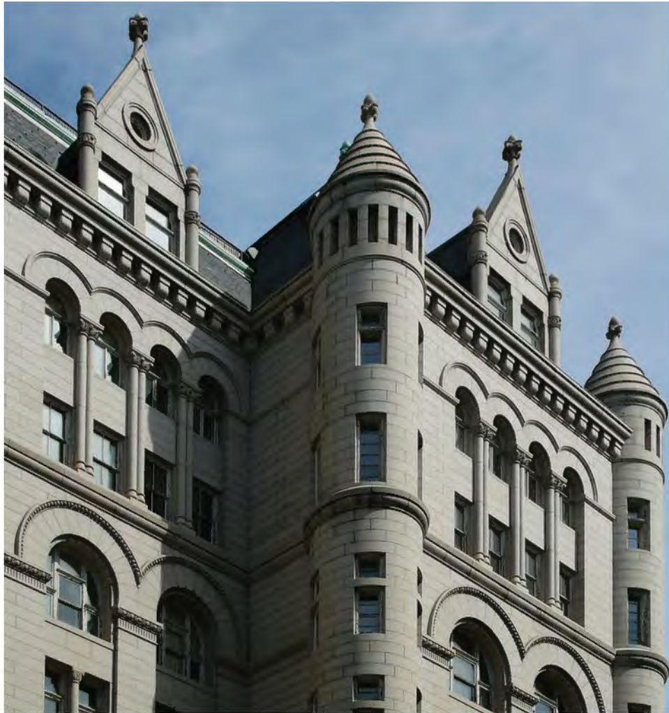
FIGURE 25: Detail of the South Elevation 6th& 7th Floor Openings, 2012. Photo Courtesy OLBN Inc.
