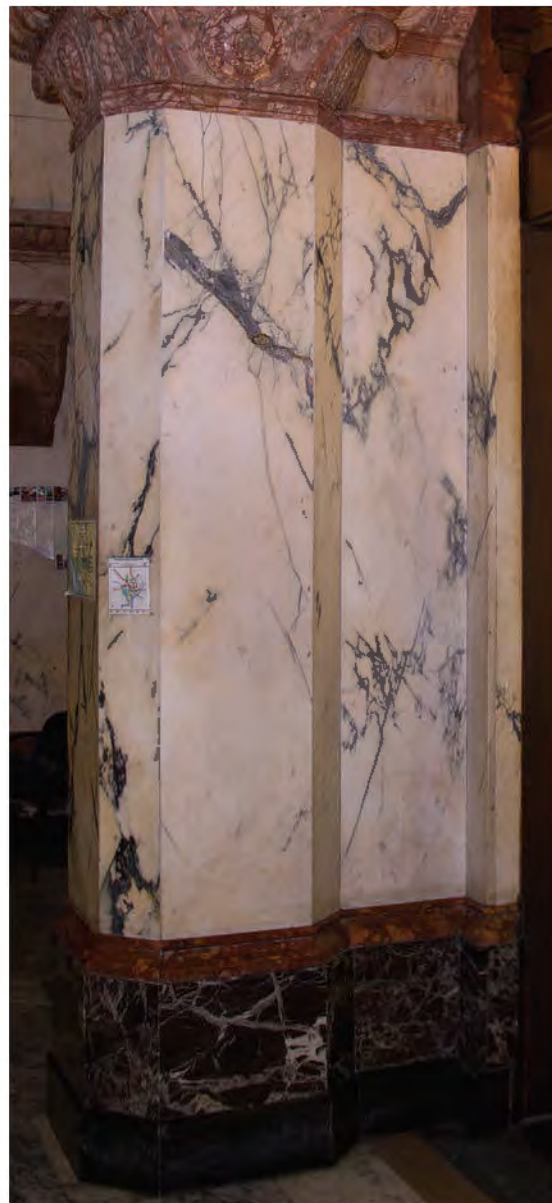
FIGURE 43: Detail of Tower Lobby South Wall Pilaster, 2012. Image Courtesy of OLBN Inc.
