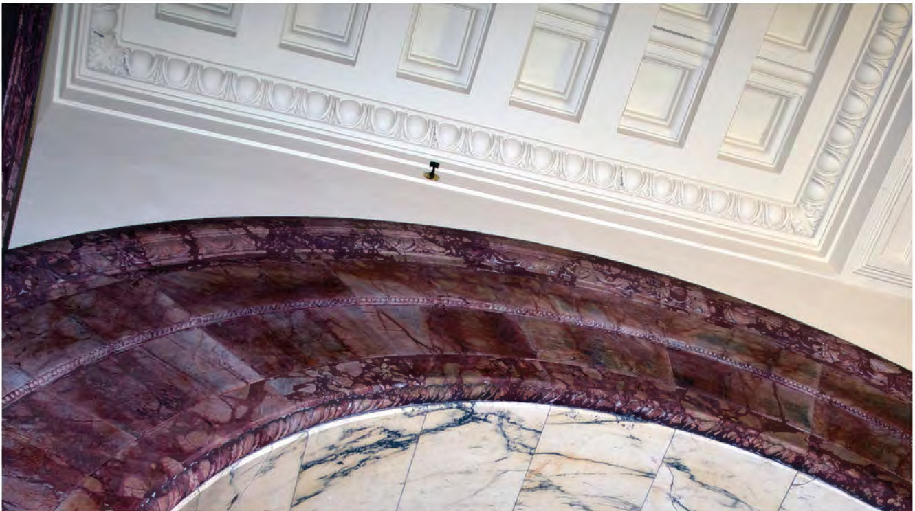
FIGURE 24: Detail of Tower Crown Moulding, 2012. Image Courtesy of OLBN Inc.
