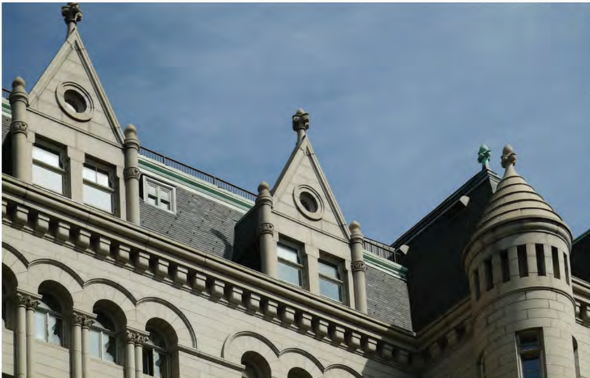
FIGURE 26: Detail of the South Elevation Cornice, 2012. Photo Courtesy OLBN Inc.
