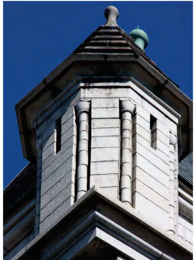
FIGURE 48: Detail of the Clock Tower Pinnacle, 2012. Photo Courtesy OLBN Inc.
