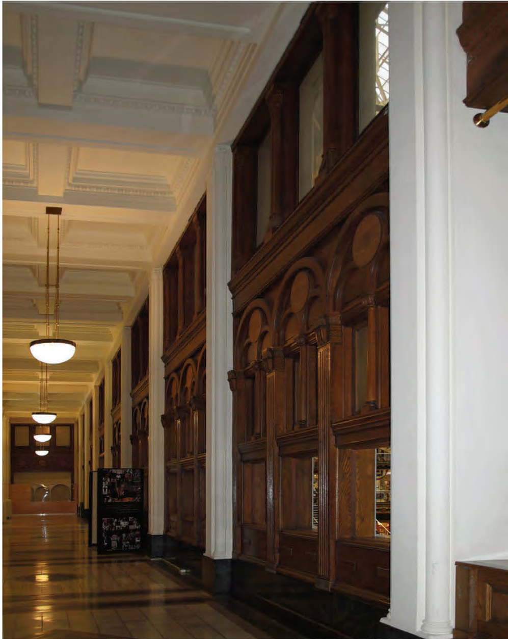
FIGURE 6: View of 11th Street Cortile Corridor Looking South, 2012. Photo Courtesy OLBN Inc.
