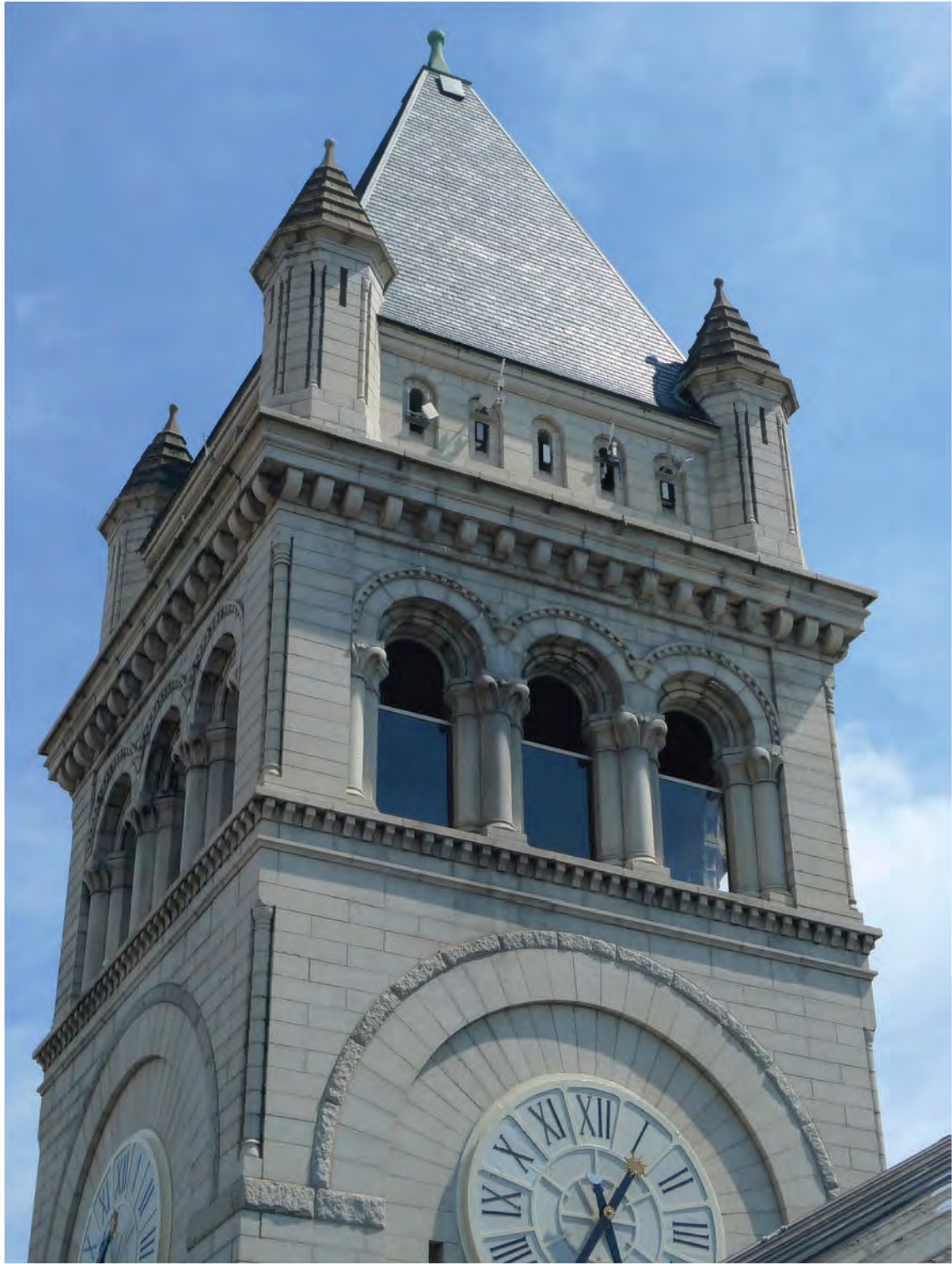
FIGURE 47: Detail of the Clock Tower NW View, 2012. Photo Courtesy OLBN Inc.
