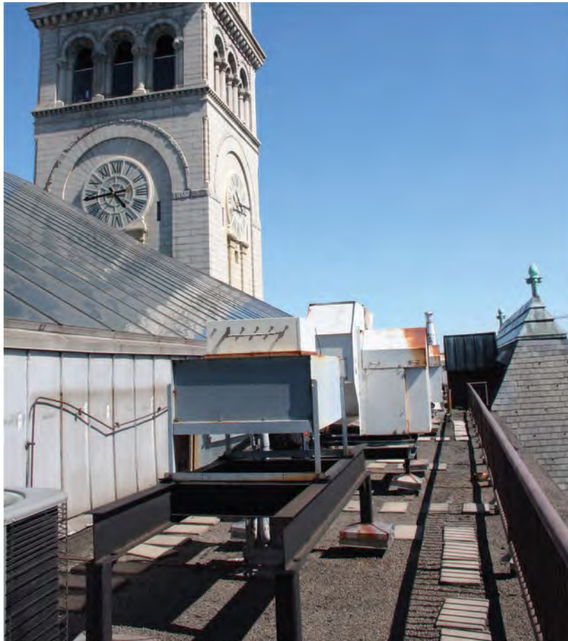
FIGURE 108: Roof, 2012. Photo Courtesy OLBN Inc.
