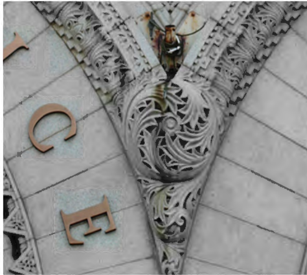
FIGURE 54: Pennsylvania Avenue Arch Label Moulding Intersection, 2012. Photo Courtesy OLBN Inc.
