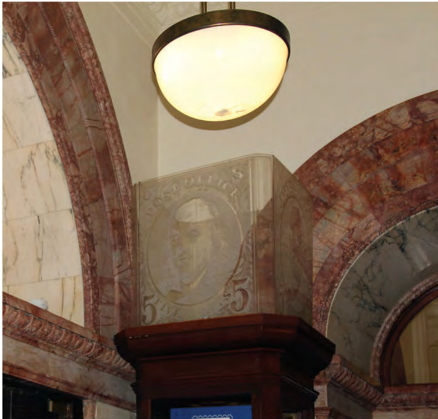
FIGURE 9: Non-contributing Elements on the Pennsylvania Avenue Entrance. Image OLBN Inc, 2012
