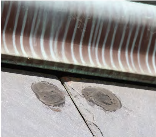
FIGURES 50 & 51: Improper Slate Repair u Face nailing the slates to the sheathing, 2012. Photos Courtesy OLBN Inc..
