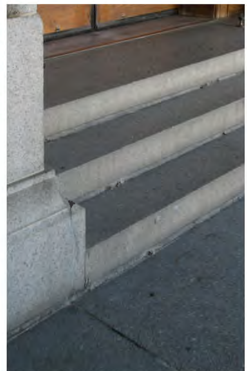
FIGURES 24, 25 & 26: Inappropriate Bituminous Joints Found Around the Perimeter of the Building, 2012. Photos Courtesy OLBN Inc.
