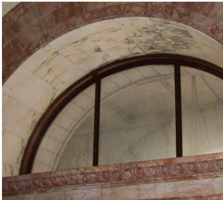
FIGURE 34: Tower Lobby North Wall Transom, 2012. Image Courtesy of OLBN Inc.
