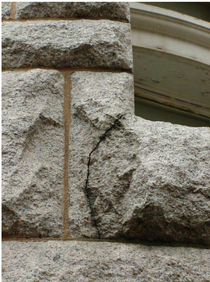
FIGURE 20: Re-pointed Joint at SW Corner Turret, 2006. Photo Courtesy T. McDowell
