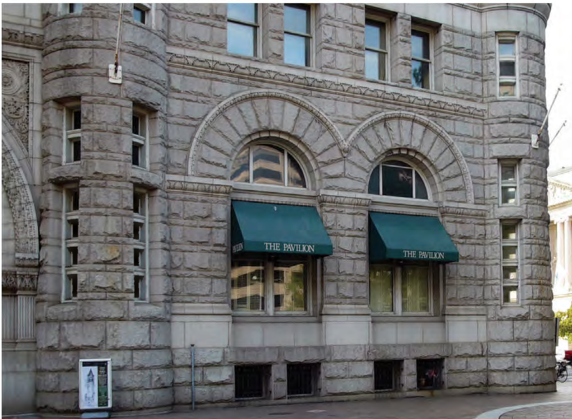
FIGURE 14: Detail of NW Building Base, 2012. Photo Courtesy OLBN Inc.
