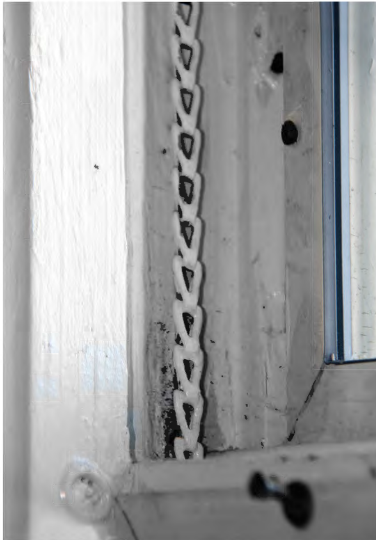
FIGURE 59: Painted Sash Chains, 2012. Photo Courtesy OLBN Inc..
