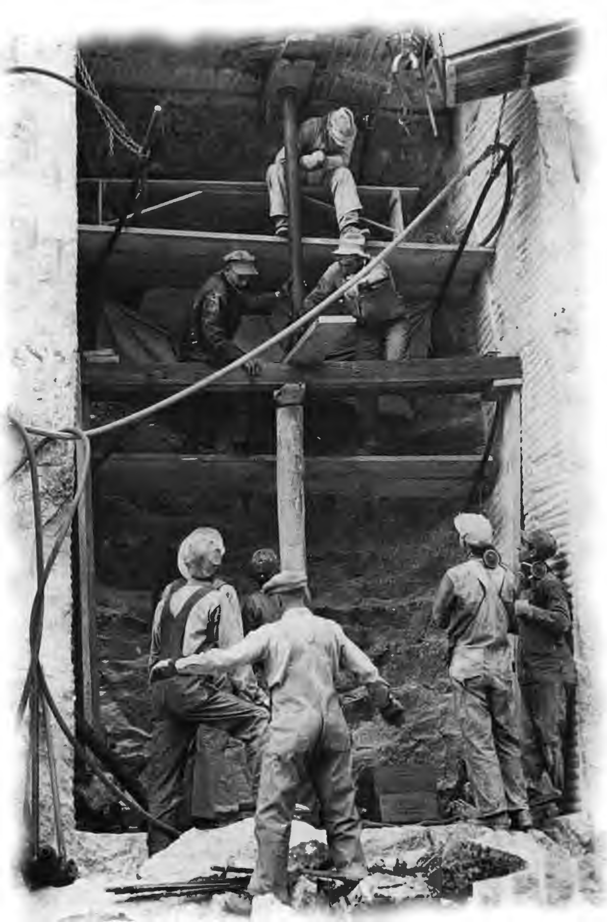
Early Hall of Records work
