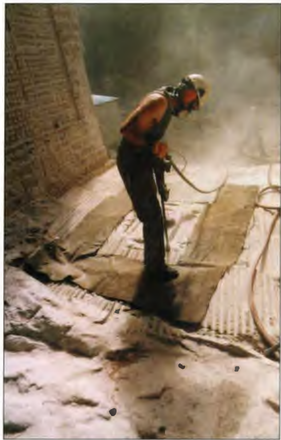
Driller Brad Johnson begins cutting the vault
