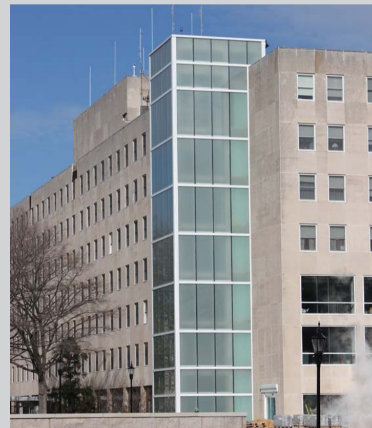
Exterior elevator located on the south end of the Sheridan building will make for easy access to the new Scott building.
