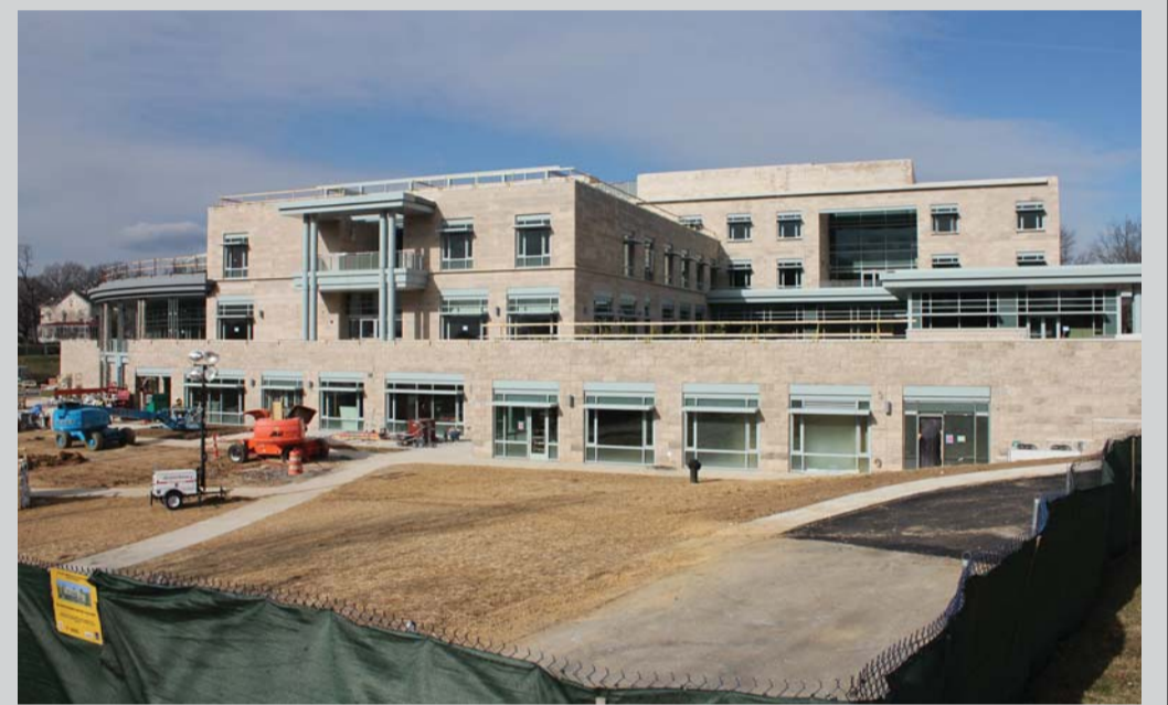
View from the rear of the new Scott building.
