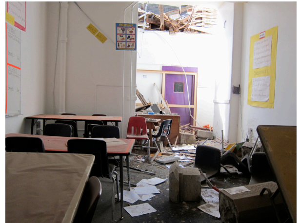
Damage under fallen chimneys, Sherman Annex and North
